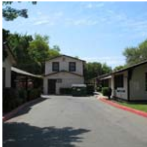
Family Shelter Before
